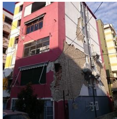
Fig. 7. Observed corner damages
