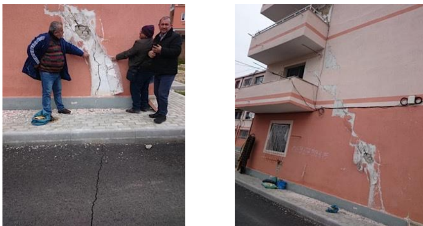
Fig. 15. Shear failure
