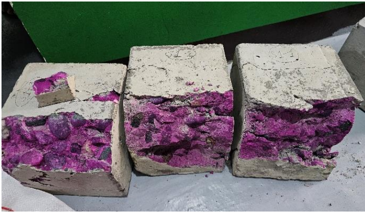
Fig. 11. Concrete samples after phenolphthalein test
