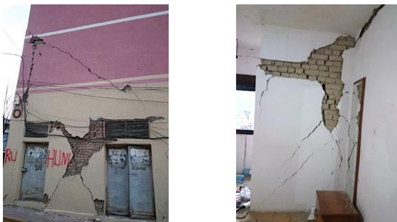
Fig. 16. Shear effect in masonry buildings
