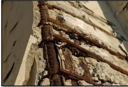
Fig. 6 Inadequate use of concrete cover [27]
