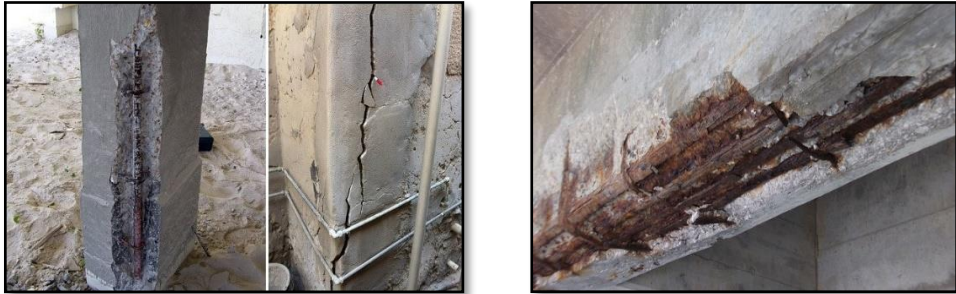
Fig. 3 Damages caused by reinforcement corrosion in columns and beams [16]
