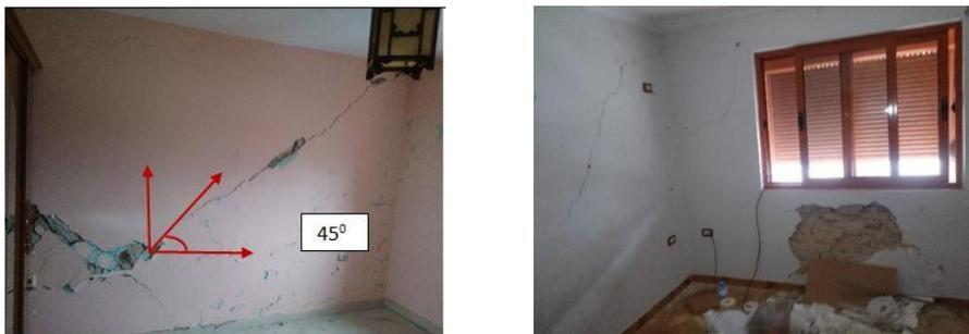
Fig. 24 Diagonal cracks extending over the height of the wall (left), spandrel damage patterns below the openings
