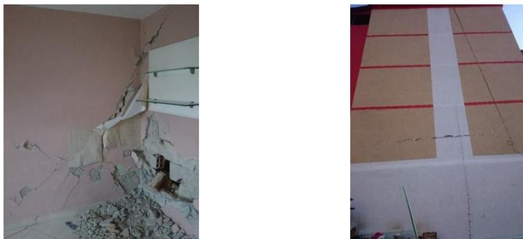
Fig. 25 Heavy cracks (more than 3 cm separation) on load bearing walls and extensive damage on non- load bearing wall (left), serious damage observed on outer facade of the building in lower stories (right)
