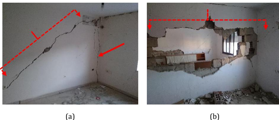
Fig. 11 (a) Extensive shear crack on load bearing wall and separation of two orthogonal masonry walls, (b) Heavily damaged partition wall in an URM building
