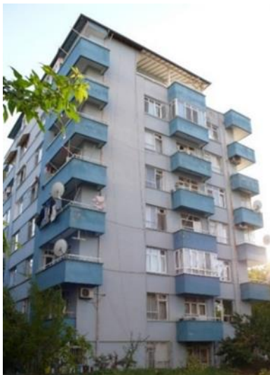
Fig. 7 The studied apartment building
