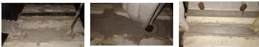
Fig. 5 Fixing of anchors and steel plate
