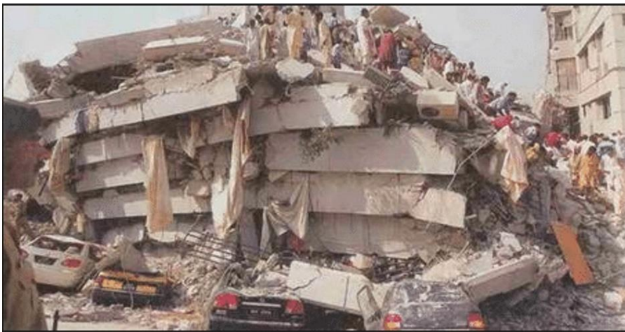
Fig. 1 Pancake failure Islamabad 2005 earthquake (Seismic design characterization of RC special moment resisting frames in Pakistan-field survey to laboratory experiments.)
