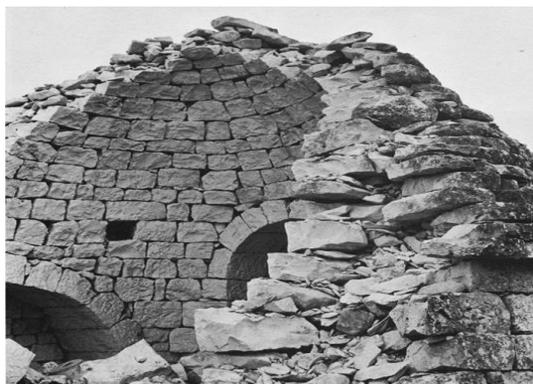
Fig. 2 Example of partial collapse of *Trullo* vault [1]
