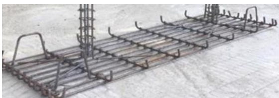
Fig. 3 Reinforcement details of raft footing
