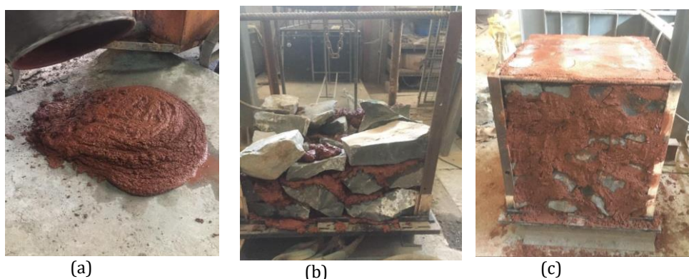
Fig 4. (a) Lime mortar, (b) Preparation of rubble masonry, and (c) final prepared rubble masonry cube
