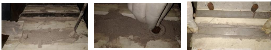
Fig. 5 Fixing of anchors and steel plate
