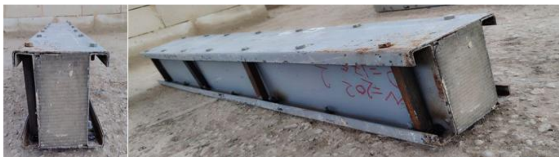
Fig. 21. Failure mode of beam BC1.15
