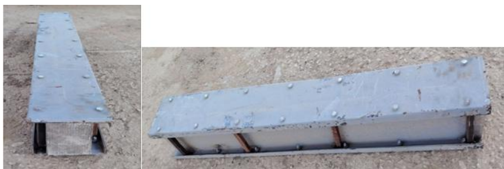
Fig. 22. Failure mode of beam BC1
