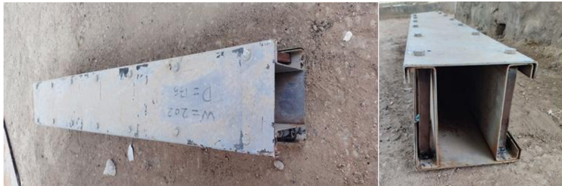
Fig. 10. Failure Mode of Beam BH1.15
