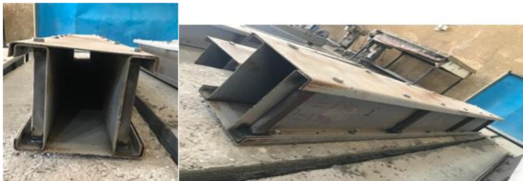
Fig. 11. Failure Mode of Beam BH1
