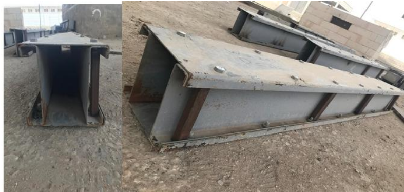
Fig. 9. Failure Mode of Beam BH1.3
