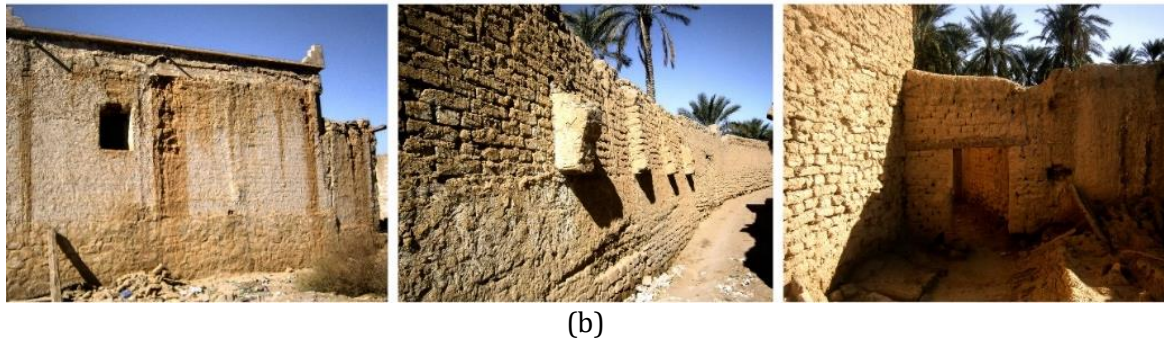
Fig. 8. Views of the wall systems in the ksar of Chetma: a) load-bearing walls (base, wall, crowning, and surface); b) construction systems of the base of load-bearing walls. Photos by authors, 2024
