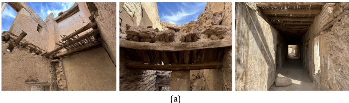
Fig. 6. Views of the wall systems in the ksar of Lichana: (a) load-bearing walls (base, wall, and top); (b) construction systems of the base of load-bearing walls (with and without stone footing). Photos by authors, 2024
