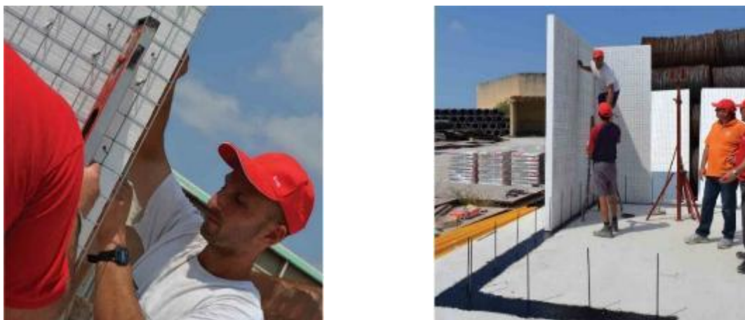
Fig. 4. Erection of wall panels [15]
