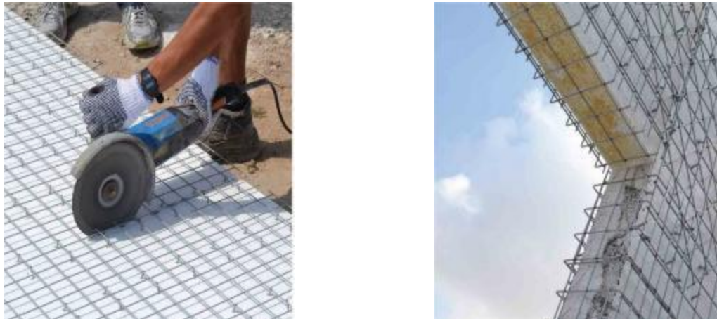
Fig. 6. Cutting method of 3D panel [15]
