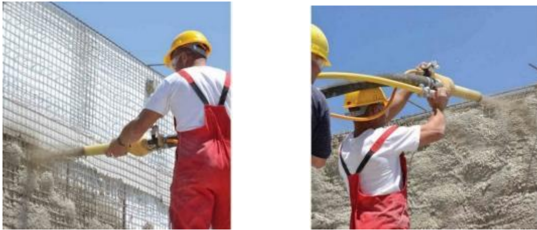
Fig. 9. Shotcrete of mortar/concrete [15]
