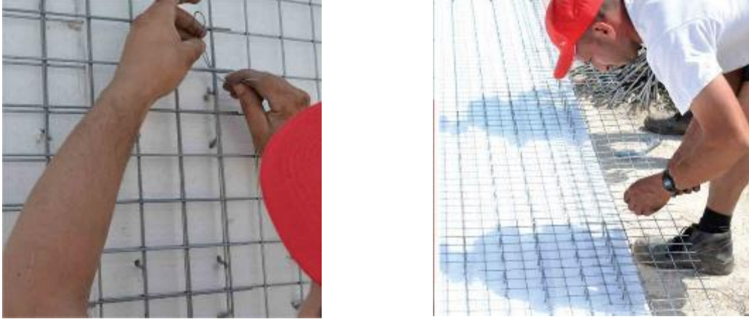
Fig.5. Reinforcing panels splices [15]
