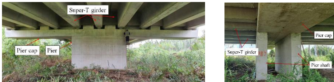
(a) Overview of investigated pier
