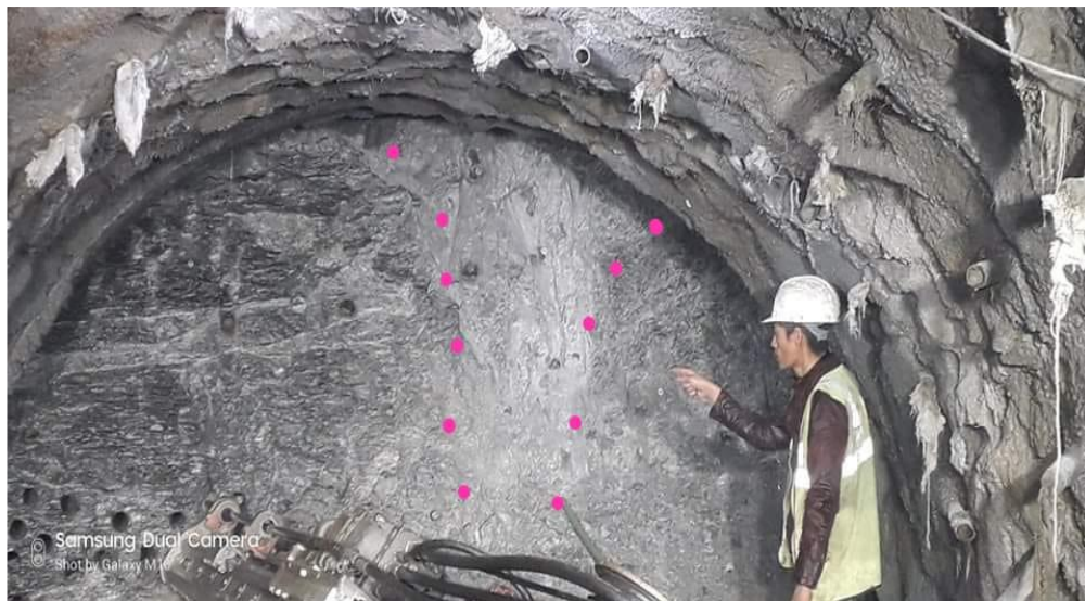
Fig. 13. Face Ch. 1+156.94 m after rectification of collapse section on June 21, 2020
