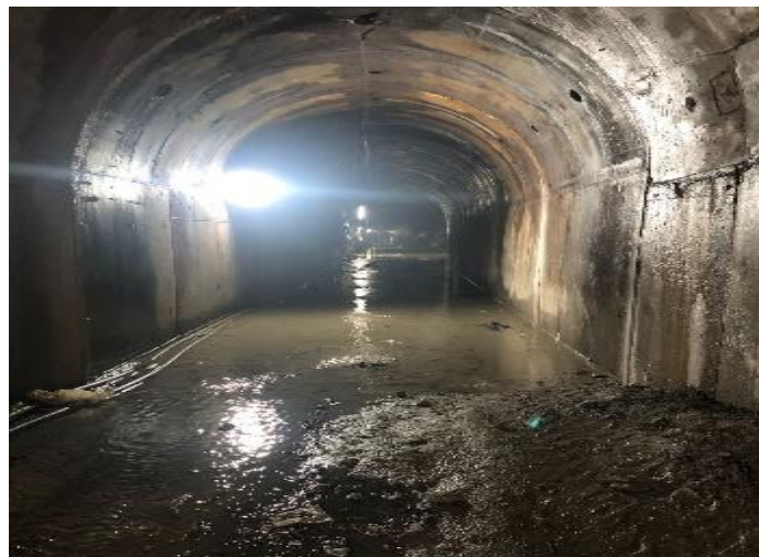
Fig. 23. Photograph of 12mm Thick Steel Liner (non-deformed)
