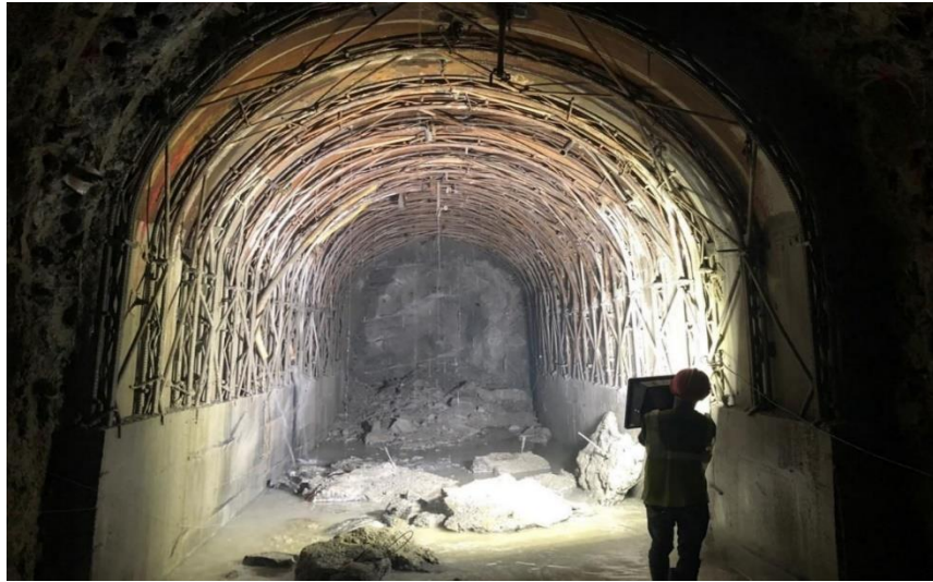
Fig. 18. Support at collapse section prior excavation resumes
