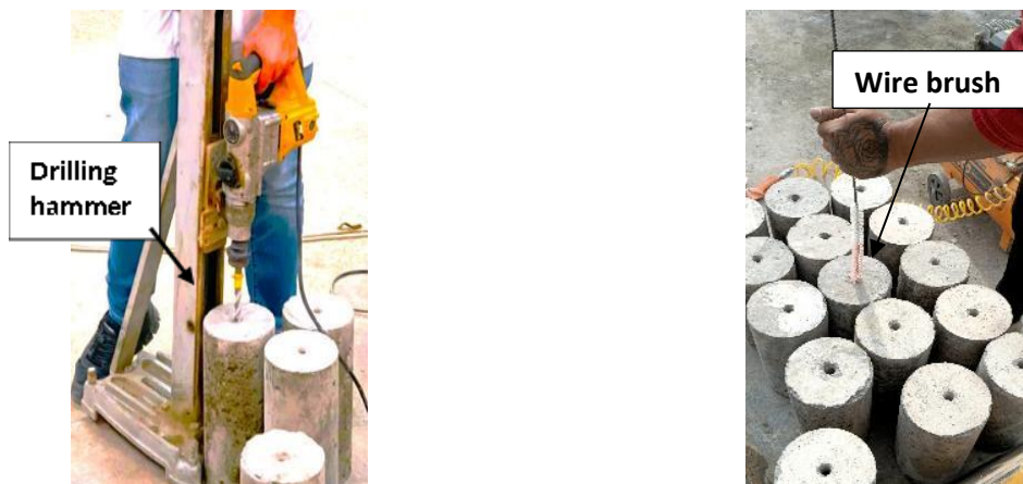
Fig. 2. Drilling and cleaning of the holes
