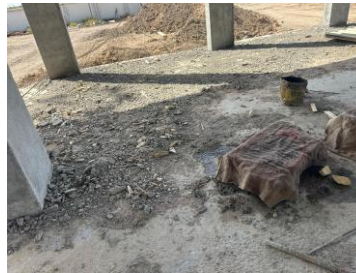
(d) Wet-burlap covering used for moist curing
