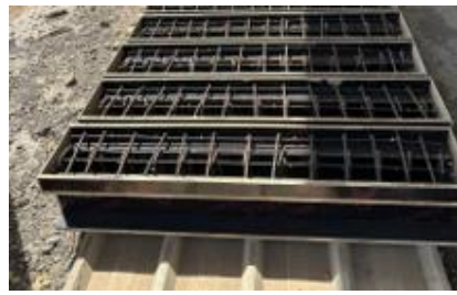
(b) Reinforcement cages before concrete placement
