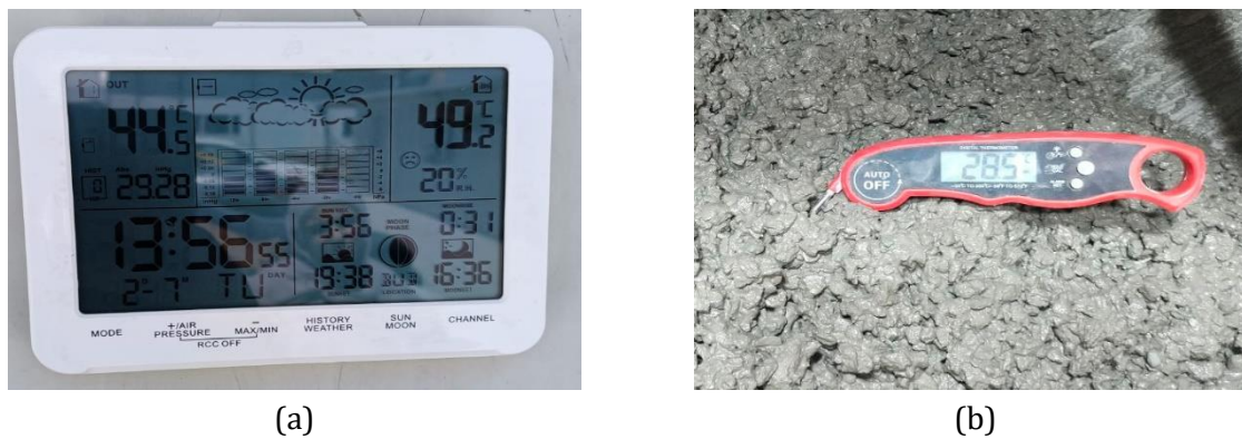
Fig. 3. The devices used to record details during casting (a) Humidity and temperature of the weather, (b) Measuring concrete temperature during mixing
