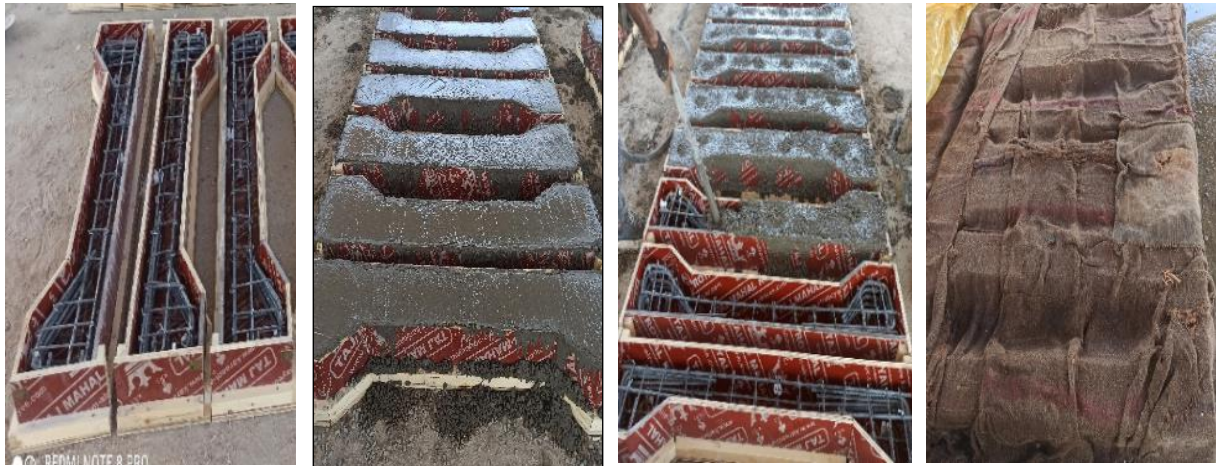
Fig. 2. Casting process phases
