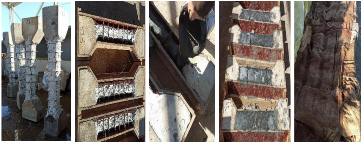
Fig. 6. Sequential steps of RC column repair
