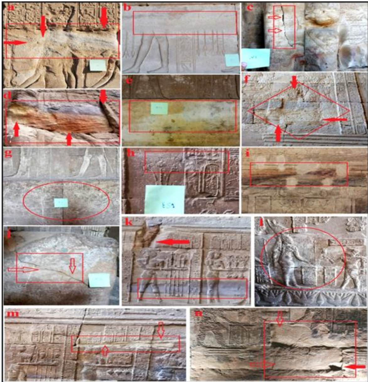
Fig. 2. (a), (b) Weathering out "granular disintegration into sand", (c) Efflorescence salts on stone surface and fissures, (d) Weathering out of stone components and coloration due to migration of iron oxides, (e)(h)(i) Efflorescence salts on stone surface, (f) Weathering out dependent on stone structure, g. Relief due to the effect of salts, (i) Coloration due to the effect of iron oxides, (j) Efflorescence salts and crack in the stone surface, (k) (m) The arrow indicates the loss of stone components and the rectangle indicates coloration due to migration of iron oxides, (n) Granular disintegration and scaling of the stone due to salt crystallization.
