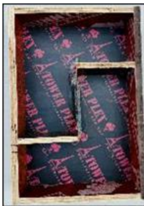
Fig. 2. Preparation of plywood formwork and reinforcement
