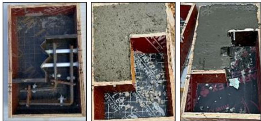
Fig. 2. Preparation of plywood formwork and reinforcement
