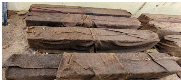
Fig. 5. Membrane curing of RC Beams
