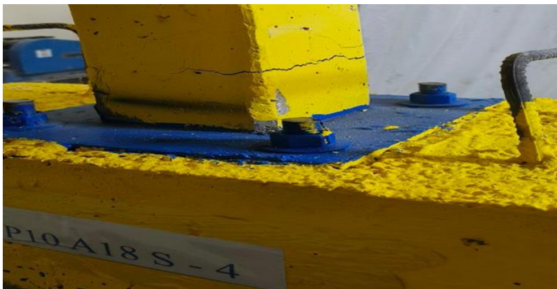
Fig. 22. Failure mode of (4 P10 A18 S -4) specimen
