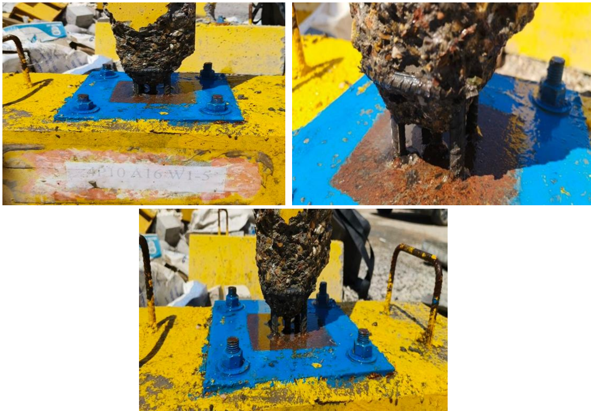
Fig. 18. Specimen (4P10A16W1-5) after removal of concrete from the contact zone between the concrete and the base plate
