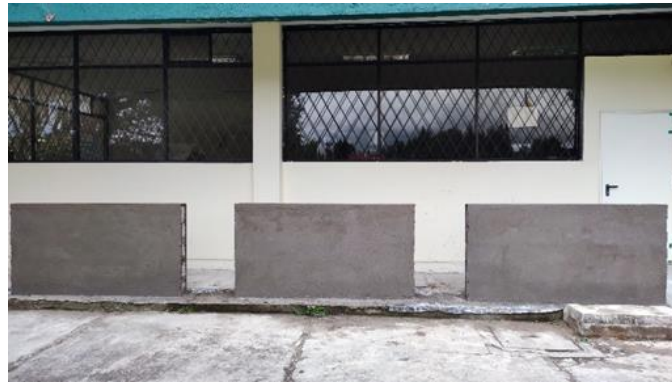
Fig. 15. Plastered Pressed Block Masonry
