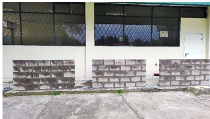
Fig. 14. Pressed block masonry
