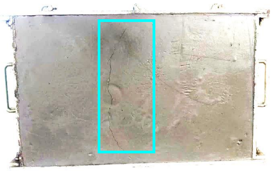
(d) Appearance of Full Crack after 12 hours
