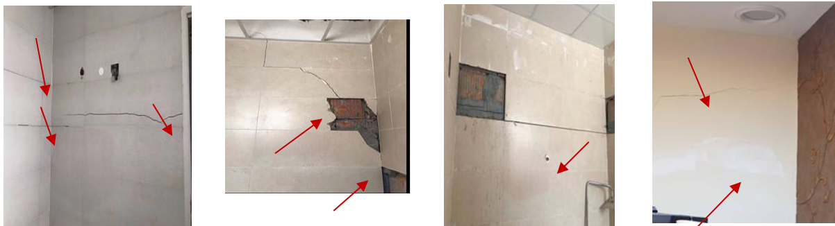
Fig. 2. Shape and position pisparate fissures in the examined residential compound in Kirkuk, Iraq
