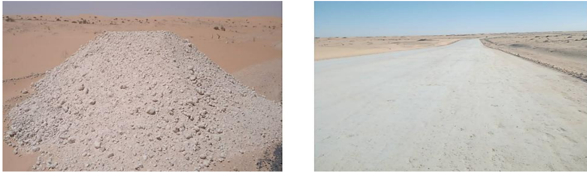
Fig. 1. Gypseous-calcareous soil before and after compaction
