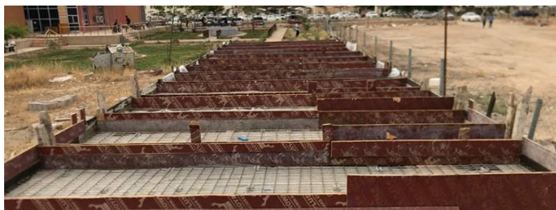
Fig. 2. Panels formwork
