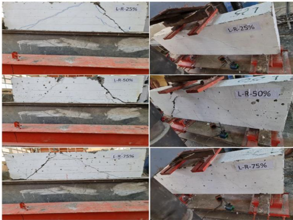
Fig. 14. Crack patterns and failure profiles of layered RAC deep beams at ultimate load stage
