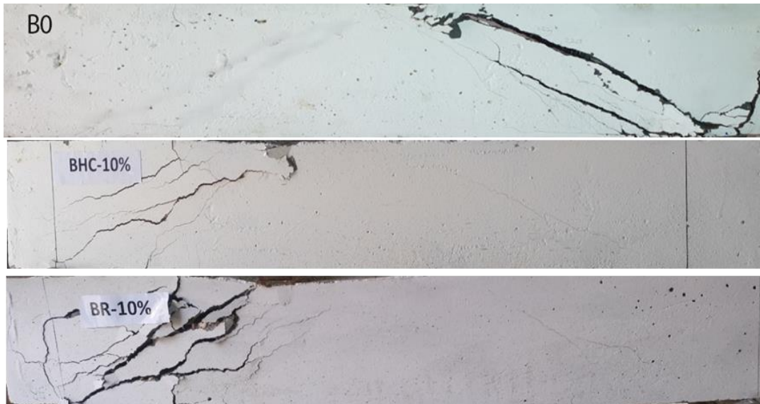
Fig. 11. Crack development of specimens B0, BHC-10%, and BR-10%
