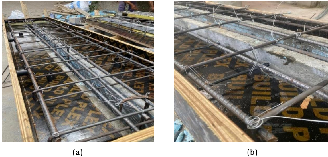
Fig. 3. Cross section of the composite beam with NWC core and UHPFRC cover, showing two plate configurations: (a) plate terminating at the bottom of the flange; (b) plate encased directly into the flange
