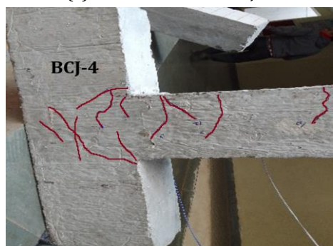
(a) Crack Patterns of BCJ-4
