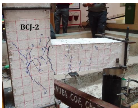
(a) Crack Patterns of BCJ-2
