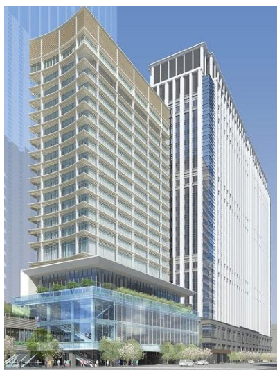
Fig. 13. The Tekko Building [197]
