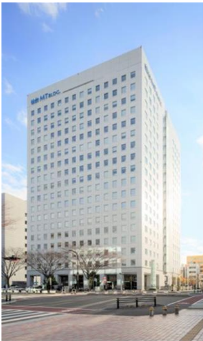
Fig. 7. Exterior View of Sendai MT [196]
