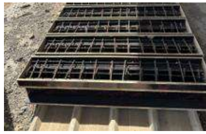
(b) Reinforcement cages before concrete placement
