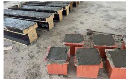
(c) Initial concrete placement and companion cube molds
