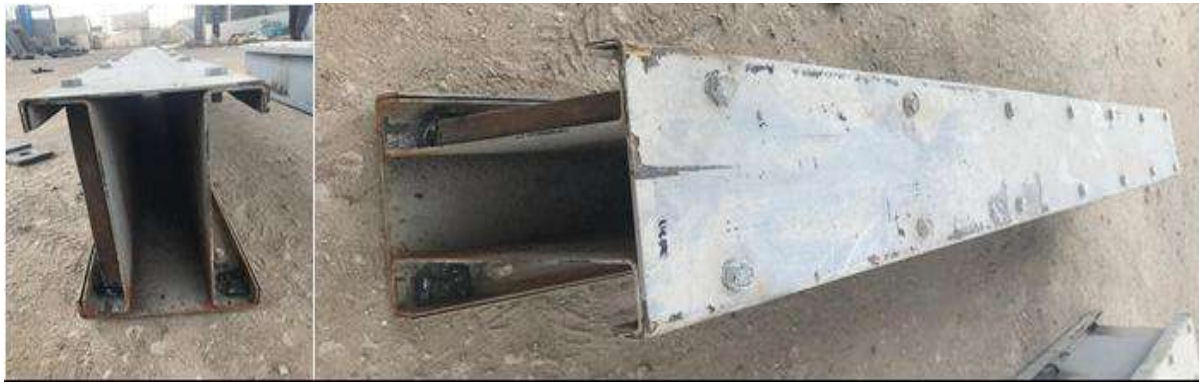
Fig 13. Failure Mode of Beam BH0.7
