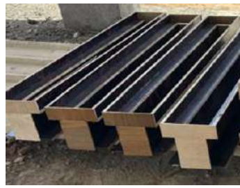
(a) Wooden formwork
