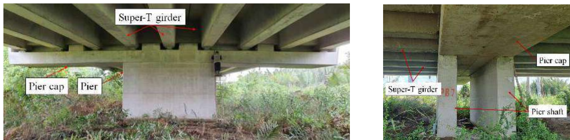
(a) Overview of investigated pier
