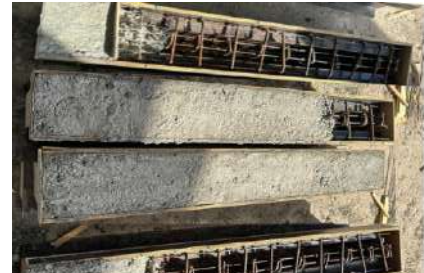
(f) Staged casting showing exposed reinforcement before subsequent placement
