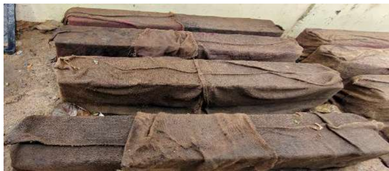
Fig. 5. Membrane curing of RC Beams
