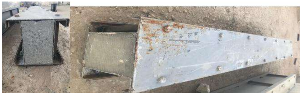
Fig. 20. Failure mode of beam BC1.3
