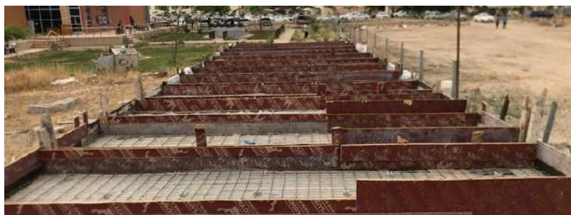
Fig. 2. Panels formwork
