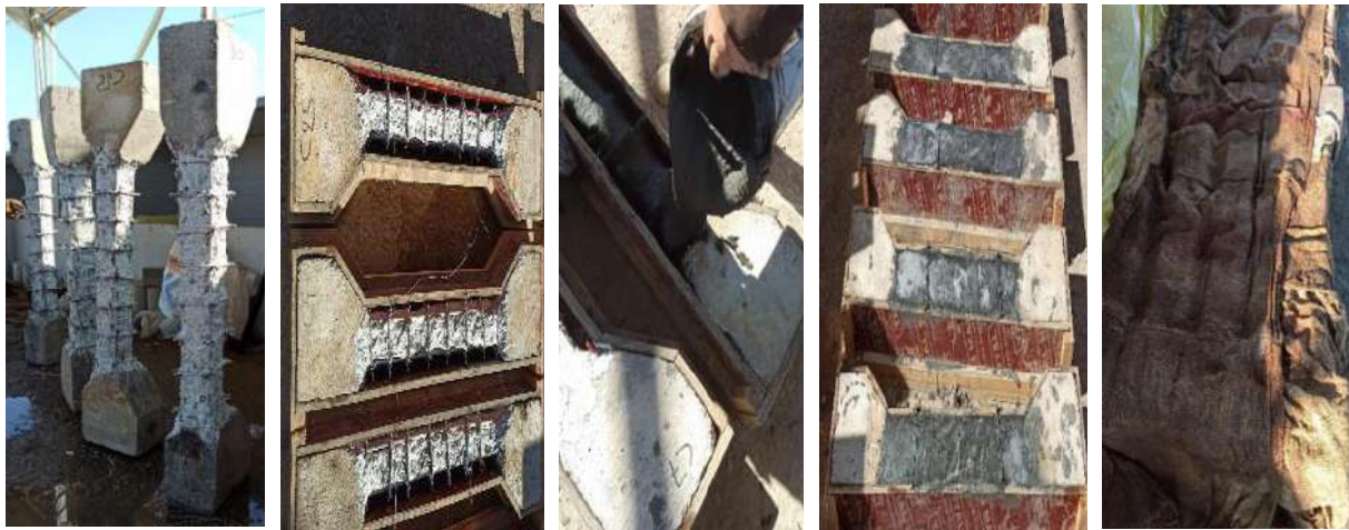
Fig. 6. Sequential steps of RC column repair
