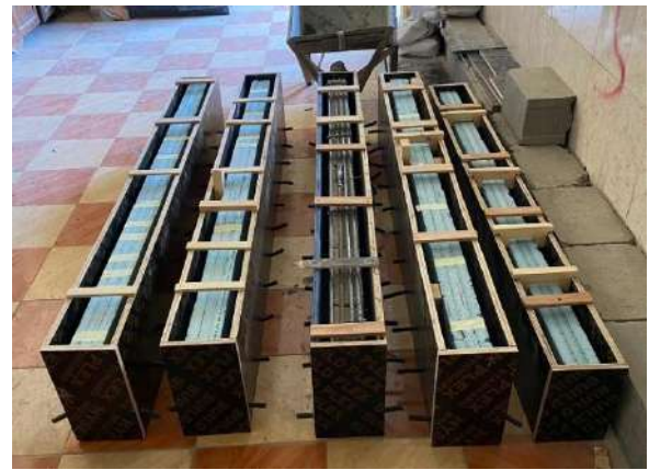
Fig. 9. Prepared inner and external formwork for all beams
