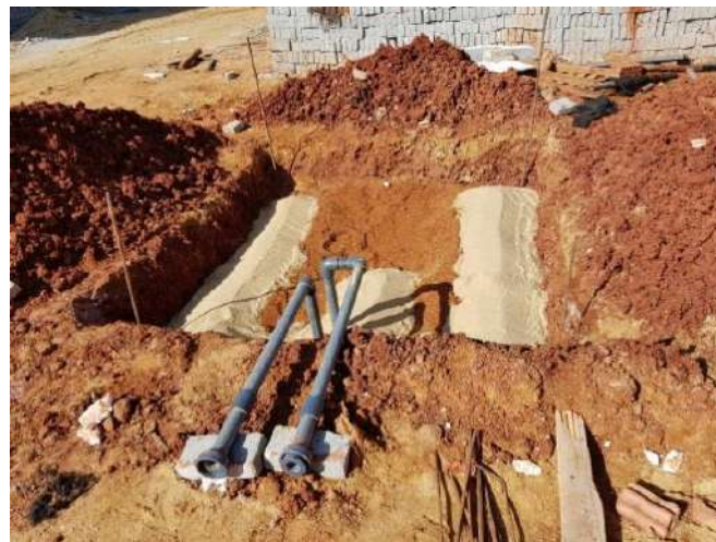
Fig. 11. A thin sand layer to prevent the settlement of pipes
