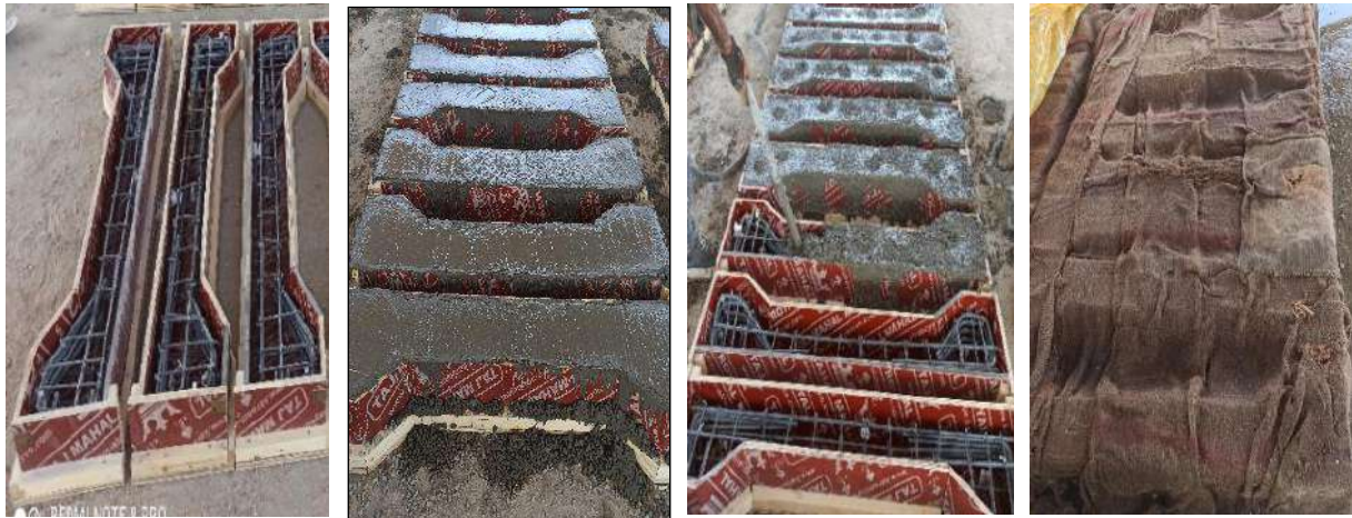
Fig. 2. Casting process phases
