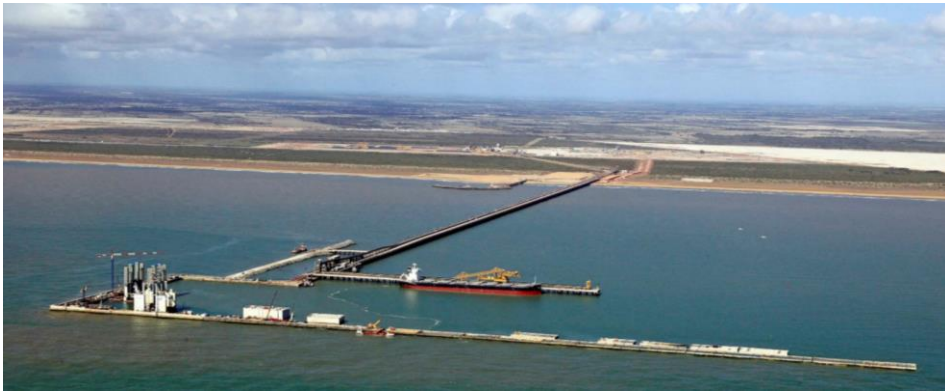
Fig. 1 View of the access bridge port complex Açú [5]
