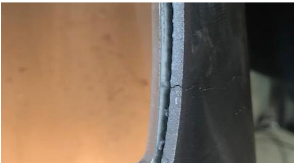
Fig. 13 Cracking in Pole Wall
