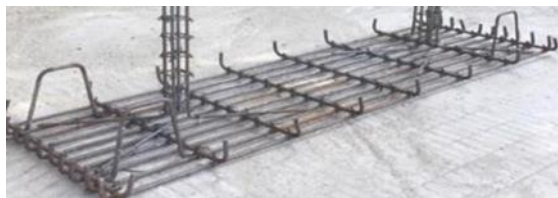
Fig. 3 Reinforcement details of raft footing
