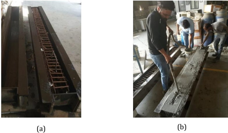
Fig. 2 (a) Reinforcement and mould for preparing the specimen and (b) Casting of specimen
