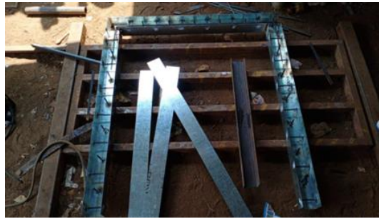
Fig 2. Welded shear connectors
