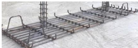
Fig. 3 Reinforcement details of raft footing
