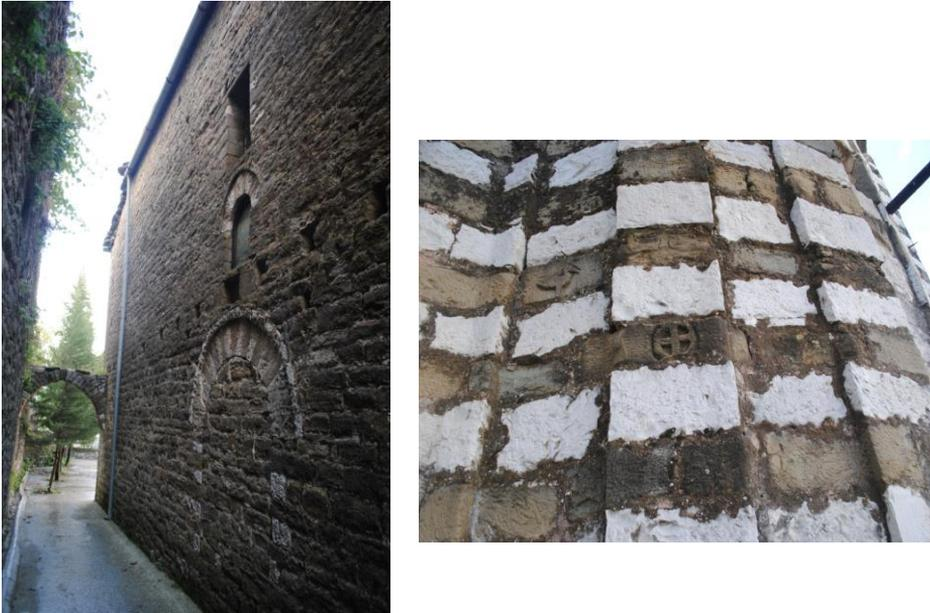
Figure 4. Western wall of the Basilica (left); Different colored stones, Eastern wall of the Basilica (right)
