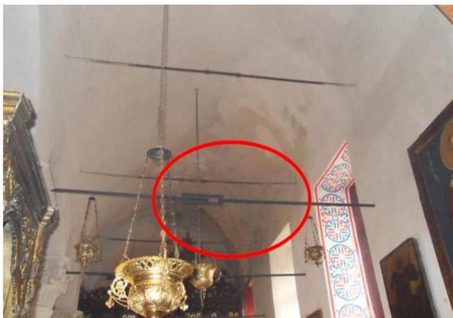
Figure 6. Barrel vault over the South aisle, moisture concentration
