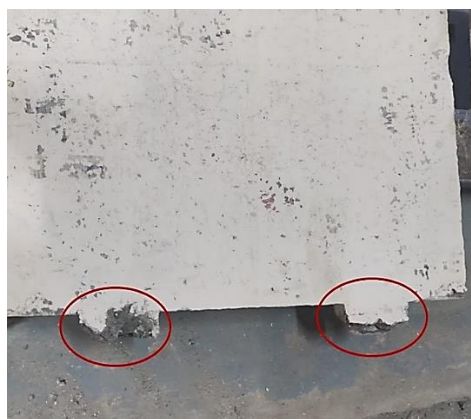
Fig. 12 Failure from RW1 specimen
