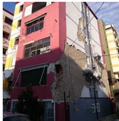
Fig. 7. Observed corner damages
