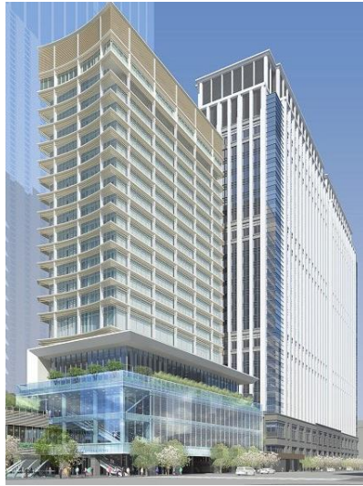
Fig. 13. The Tekko Building [197]
