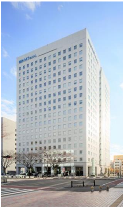
Fig. 7. Exterior View of Sendai MT [196]
