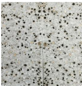
Fig. 10. Fractured LWC after split tensile test
