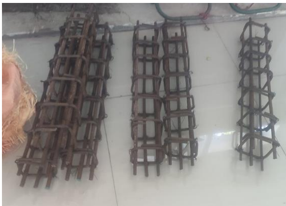
Fig. 4. Rebar arrangement in the cage
