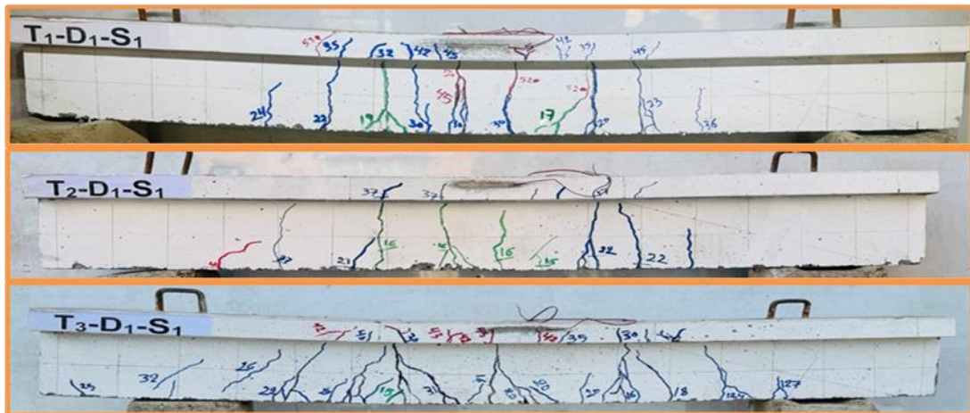
Fig. 11. Crack patterns and failure modes for T-beams reinforced with steel bar of 8 mm
