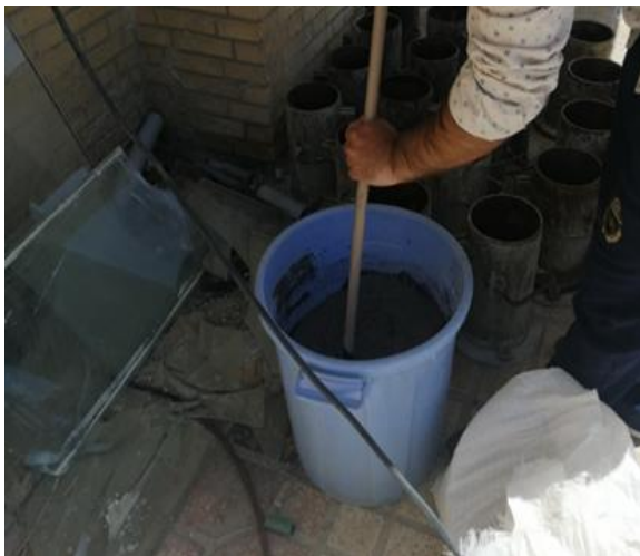
Fig. 1. Adding water to bentonite and preparation for making concrete
