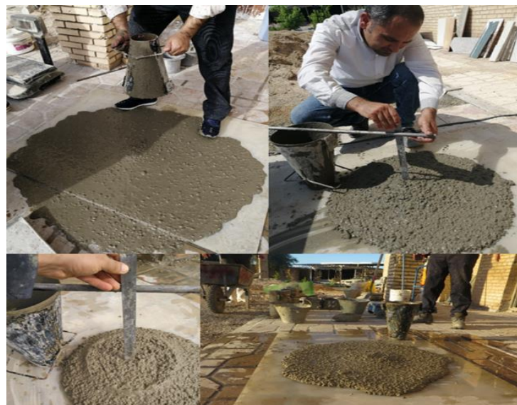
Fig 4. Slump test: (a) flowability of plastic concrete with carbon, (b) height difference of plastic concrete with slump, (c) determination of slump of plastic concrete with carbon and (d) efficiency and fluidity of plastic concrete with carbon on a flat plate
