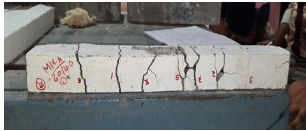
Fig. 10. Crack patterns of the specimen
