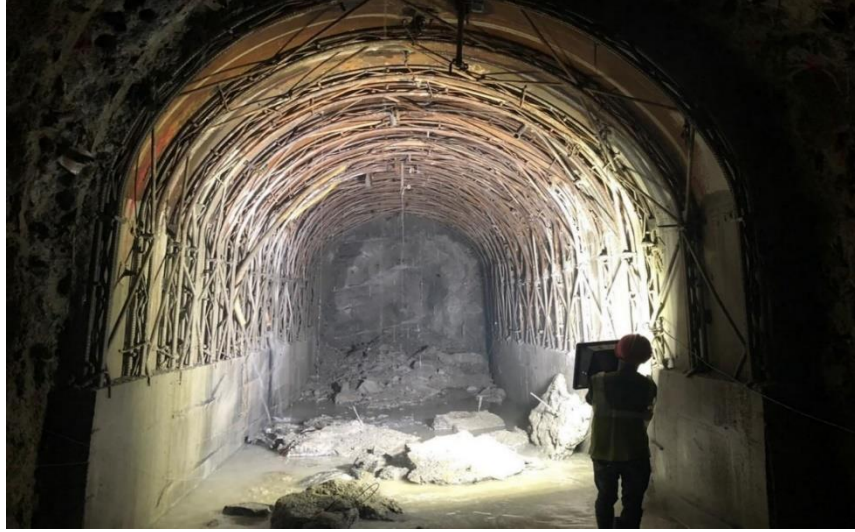
Fig. 18. Support at collapse section prior excavation resumes
