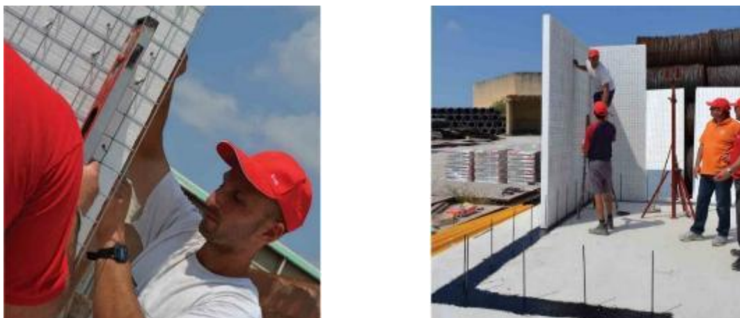
Fig. 4. Erection of wall panels [15]
