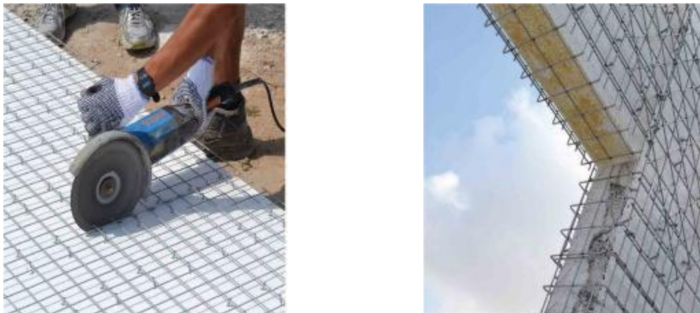
Fig. 6. Cutting method of 3D panel [15]
