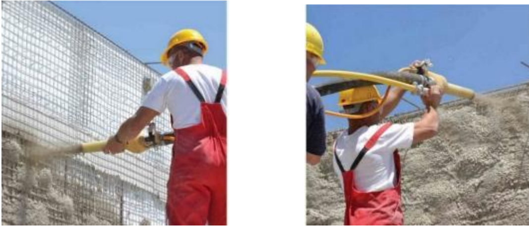
Fig. 9. Shotcrete of mortar/concrete [15]
