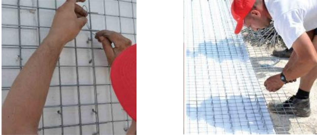
Fig.5. Reinforcing panels splices [15]
