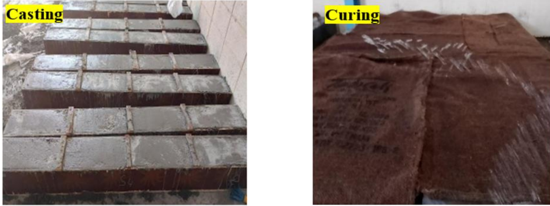
Fig. 1. Casting and curing of beams
