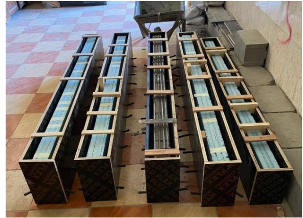
Fig. 9. Prepared inner and external formwork for all beams
